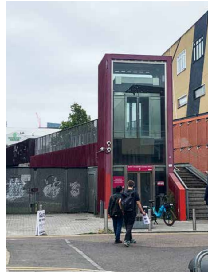
Fig 5.26 Public lift at Hackney Wick, London
